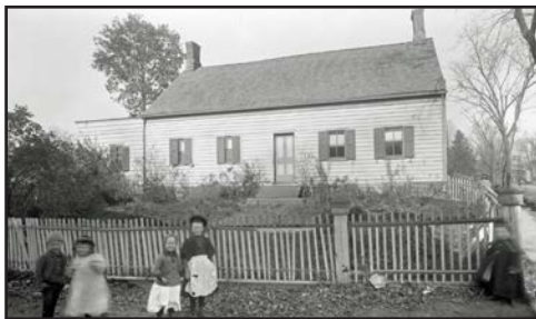
The Daniel Dodd House 339 Franklin Street: Demolished
