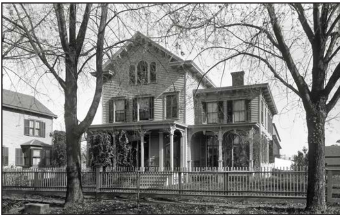
15 Spruce Street: Demolished
