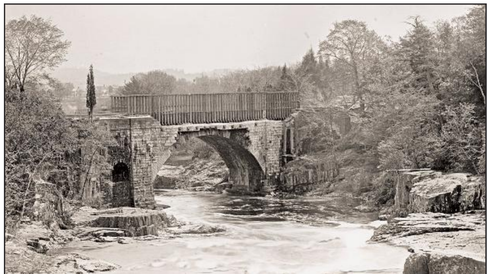
The Morris Canal aqueduct over the Passaic River in Little Falls, NJ was constructed of brownstone from a quarry a short distance downstream. Completed in 1829, the aqueduct was blasted to pieces in 1925. Its destruction was considered by Alvin Harlow, a canal historian, to be "an act of violence."
