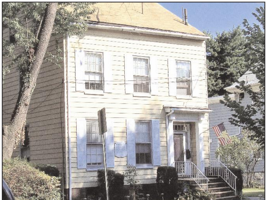
The Hall House on Oakland Avenue.
